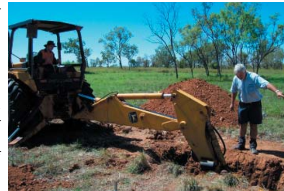
Digging Footings for Antenna Guy Wires
