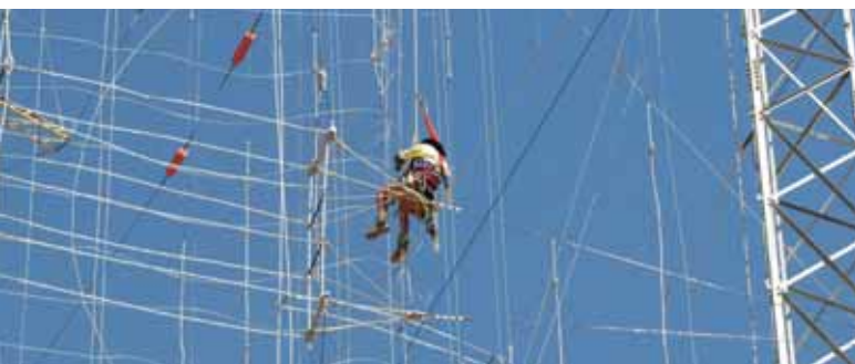
One of our resident "spiders", Chris Webb (our electrician), in his element connecting wires on a reflector screen!
